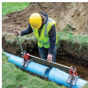
PPJ and PPJVS in use on gasketed pipe
